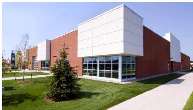
Delta College Technical Trades & Manufacturing Complex
